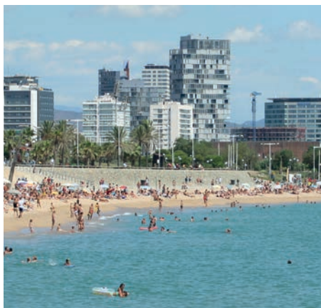
Diagonal Mar buildings
