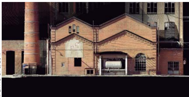
Elevation of the boiler room obtained using terrestrial laser scanner, Faro Focus 3d, produced by the Laboratori Virtual de Modelització de la Ciutat. Exterior and interior view of the point cloud.
