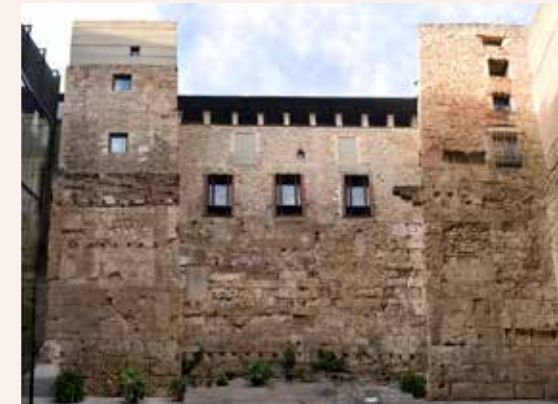
Towers and a section of the Roman wall from the late 3rd century. The upper part and the facing show the alterations made during the medieval period. © MUHBA/Pep Parer
