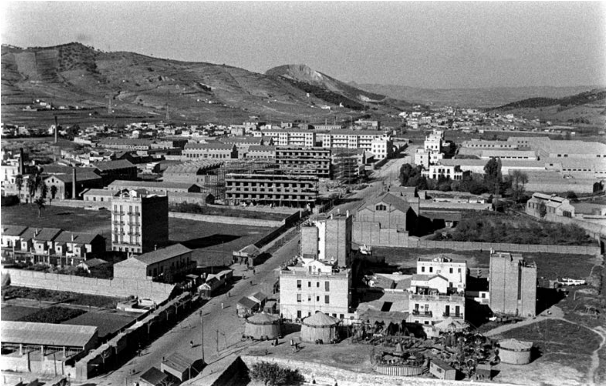
Panoramic view of Sant Andreu with Casa Bloc under construction, 1934. Margaret Michaelis. AFB
