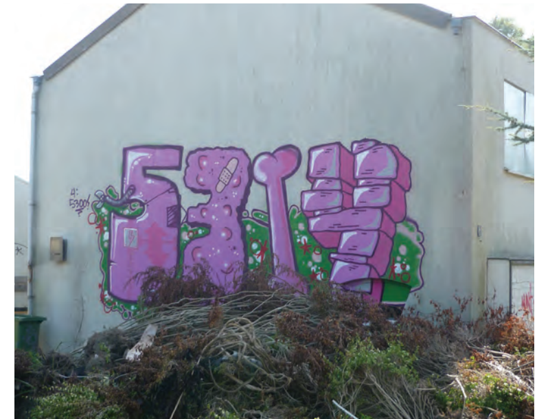
Houses in a Rotterdam-South neighborhood that are to be demolished. This area has become a favorite place for “5314” pieces. The graffiti range from detailed pieces to short, messy tags. Photo: Hans Walgenbach
