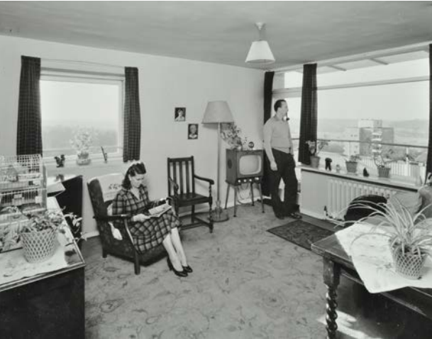
↑ London County Council, Alton Estate, Roehampton. 1952-1958. Interior of a flat. 1960. LPA
