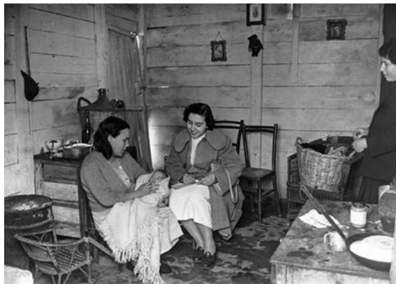
← The absence of a resolute housing policy meant that shanties were the only homes available to many families. Inside a wooden shack in Somorrostro. 1940s. Unknown photographer. CPFC
