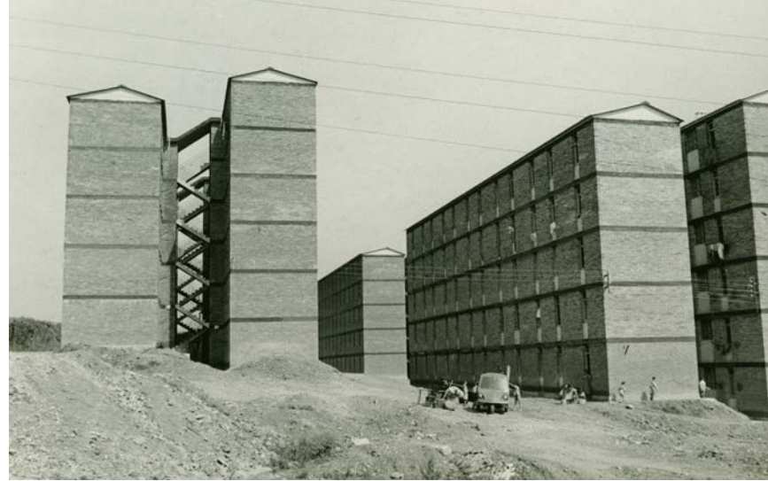
← Trinitat Nova: twin buildings in the Municipal Housing Board's second stage. 1959. Brangulí. AFB
