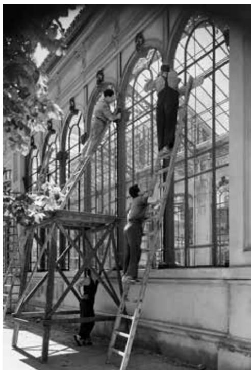
A group of Cubiertas y Tejados workers doing the preparatory work for the restoration of the Hivernacle in the 1950s.
